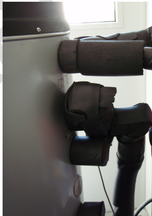
Fig. 3: Solar circuit and domestic water connection
